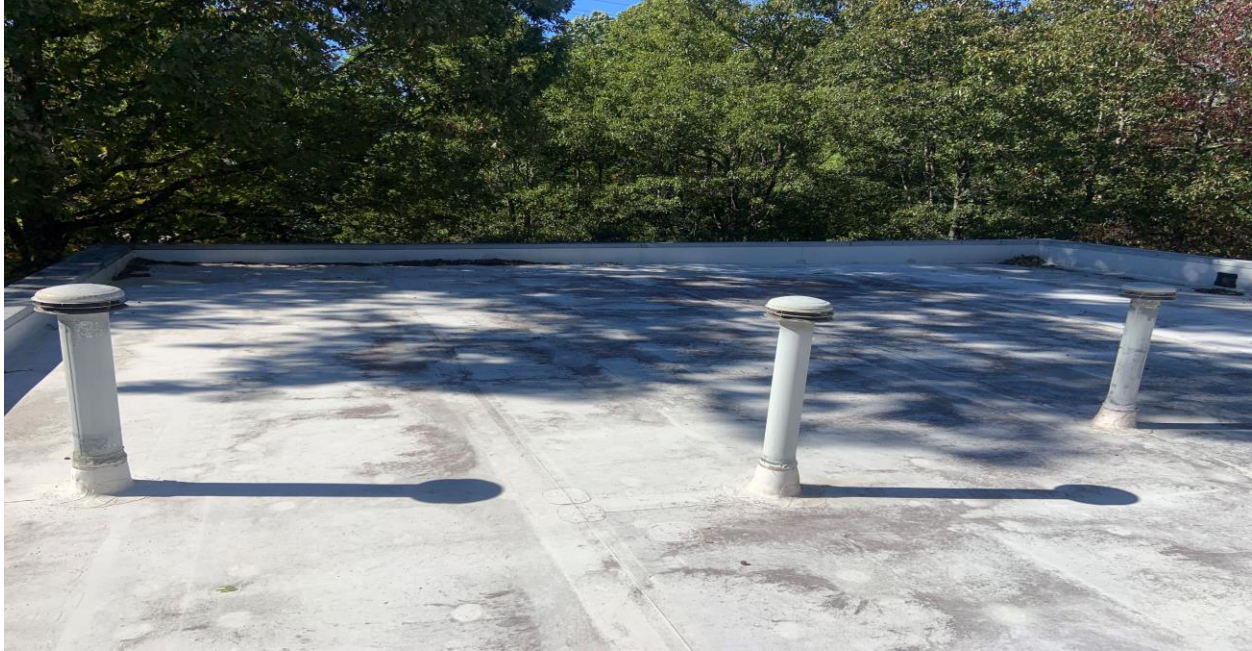
Existing TPO Roof System
